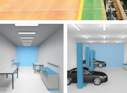
In production halls with standard hight of the walls it is suitable to use linear luminaires with the direct characteristic of the luminous flux. To obtain the standard stated levels of the maintained illuminance it production halls with non standard hight of the walls (6 m and more) it is important to choose luminaires that can be used in different mounting hight
