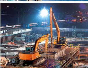
The appropriate illumination can improve the employees' sense of orientation and simultaneously reduce the risk of collisions when motor vehicles and machines move around the construction site. From the point of view of navigation it is suitable to place the identification and orientation lighting to the communication zones. The drivers' attention can be drawn to the risk zones and the necessity to slow down by using the dynamic light signals.
