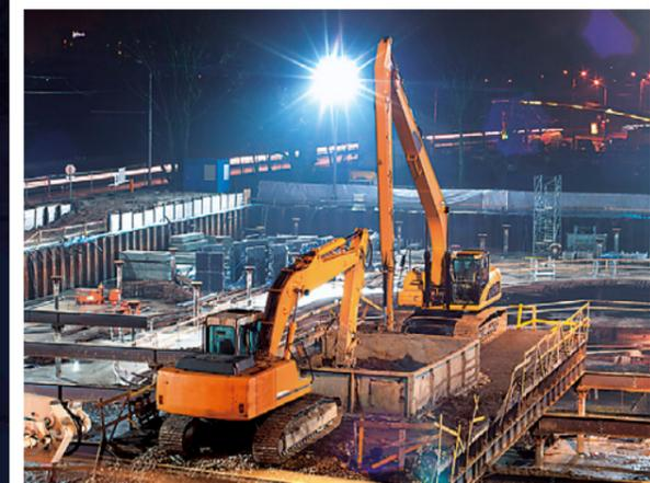
The appropriate illumination can improve the employees' sense of orientation and simultaneously reduce the risk of collisions when motor vehicles and machines move around the construction site. From the point of view of navigation it is suitable to place the identification and orientation lighting to the communication zones. The drivers' attention can be drawn to the risk zones and the necessity to slow down by using the dynamic light signals.
