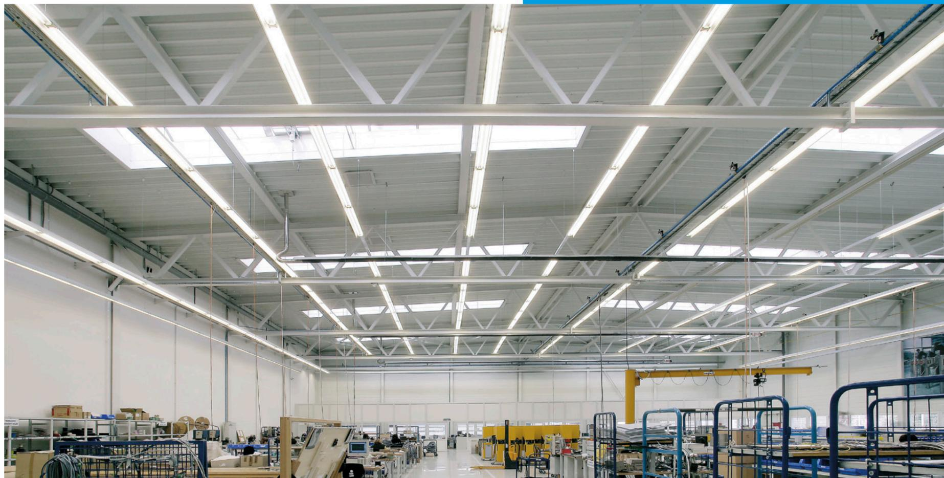
The daylight simulation is often implemented with the daylight sensor that assesses the lighting intensity in the room during the day and according to this it increases or reduces the luminaire output in the light system. In this way constant illuminance of the space in compliance with the standard is ensured during the whole day.
