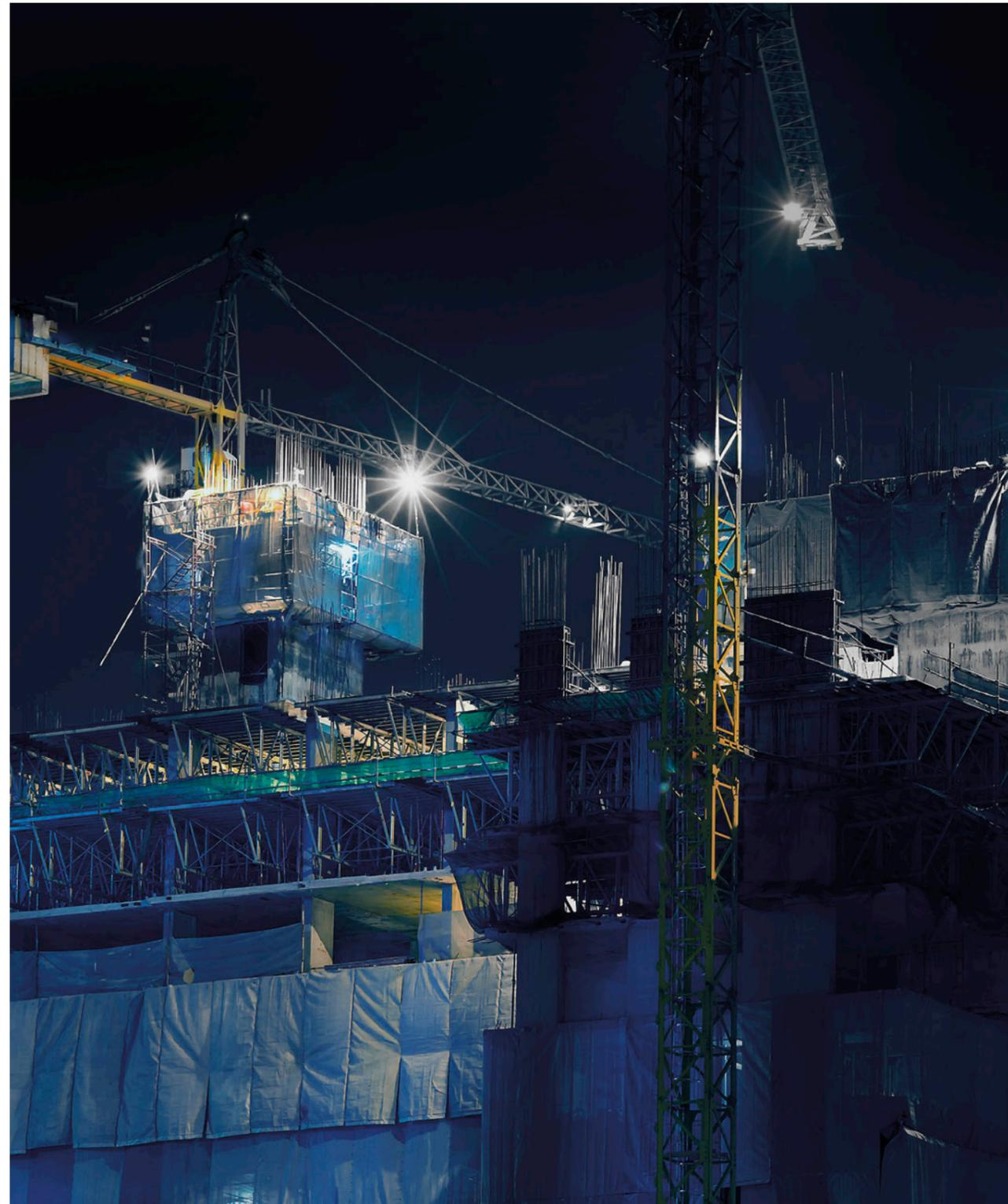
optimal lighting conditions it is suitable to install the luminaires with a wide lighting distribution curve directly to the tower and jib of the crane. When placing
